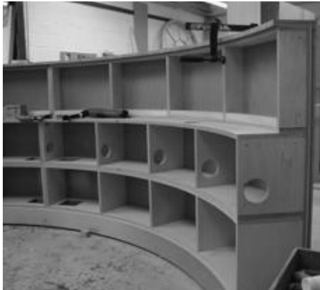
Reception desk being fabricated
